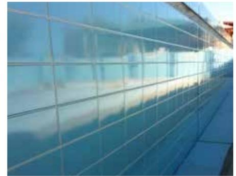
**PROJECT INFO:** A 300m<sup>2</sup> commercial pool refurb project in Barcaldine, QLD. The refurbishment of an existing 25m concrete pool shell tiled with ceramic gloss tiles.
