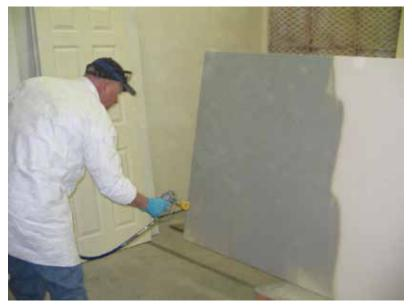
dried to a uniformolive green colour, approximately 45 to 90 minutes at  $21^{\circ}$ C, visually inspect the coating for any voids or pinholes. Fill any defects with additional material and apply the second coat at right angles to the first. The wet film thickness should be checked periodically using a wet film gauge. Each wet coat should be 0.4 - 0.6 thick. The combined dried coating should be 0.5 - 0.8 mm thick.
