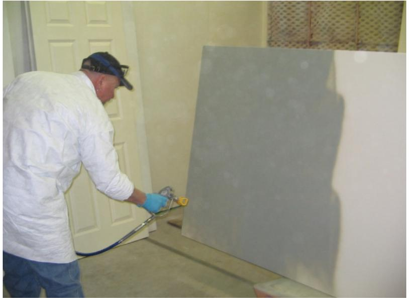
Check application thickness with a wet film gauge periodically as the HYDRO BAN is being dispensed to ensure that the appropriate thickness and coverage is achieved. Bounce back and overspray will consume more product. To achieve the required film thickness, the coating must be free from pinholes and air bubbles. Do not back roll coating. Allow the HYDRO BAN to cure in accord with the instructions in Data Sheets DS-1036 and TDS1003 prior to the installation of the tile or stone finish.
