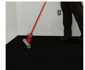
**STEP 3:** Roll GenieMat RST reduced sound transmission mat with a 16kg inoleum roller
