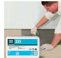
**STEP 4:** Apply polymer fortified thinset to GenieMat RST reduced sound transmission mat using an appropriate square notch
