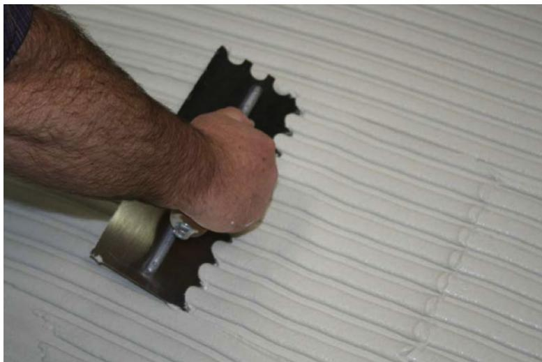
Picture 1.2 – 18 mm loop notch trowel with a medium bed adhesive used for large format tiles or stones. Trowel thin set adhesive in one direction holding trowel at a 45 degree angle. Notice the full ribbons of adhesive that left behind.
