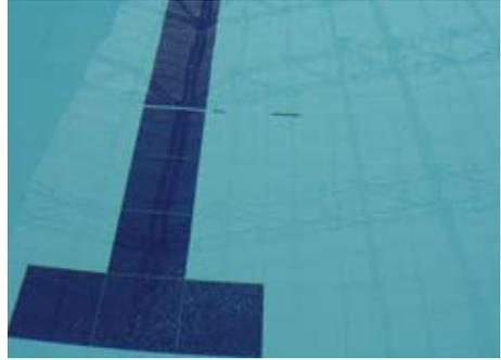
Figure 12.12 – Sealant in the movement joint is missing. In order for the sealant to maintain its functional ability, the joint must be correctly designed. Namely:
