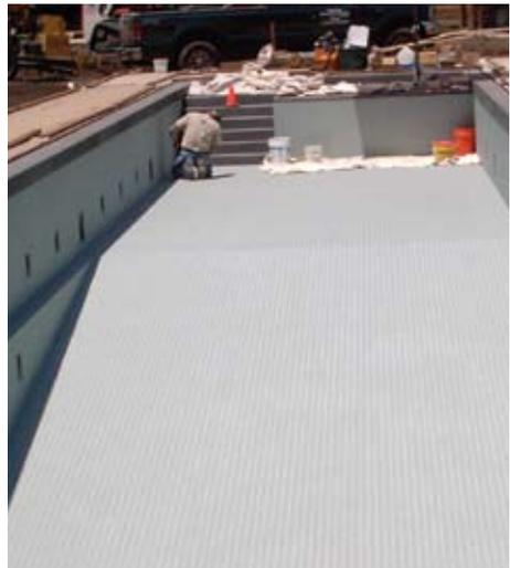
Figure 3.2 – Tiled steel pool shell.
