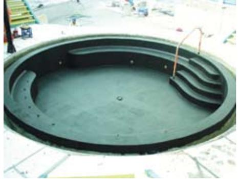
**Case Study 8** – The waterproofing installation is complete. The waterproofing membrane must be allowed to fully cure prior to the flood test. Full cure rates will vary by product type. Consult with the waterproofing manufacturer for full details.
