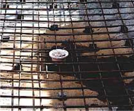
Figure 4.4 – Typical drain position and steel reinforcement prior to gunite application of concrete.
