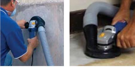
Figure 6.2 – Saw Tec® Dustless Grinding. This method is ideal for spot preparation and solves localized problems.
