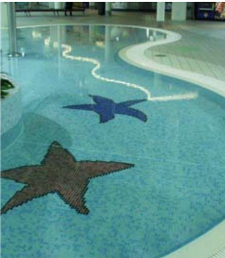
Figure 4.1 – Indoor water park wading pool with clearly defined movement joints.
