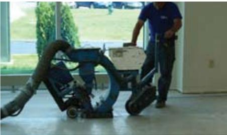
Figure 6.3 – Shot-blasting is ideal for areas outside of pool tanks and water features and for areas where access by the equipment is not an issue.
