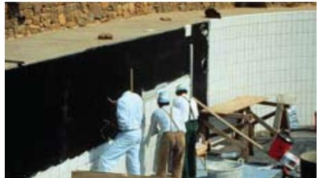
Figure 7.13 – Installation of mosaic tile with liquid latex fortified portland cement thin-set mortar.
