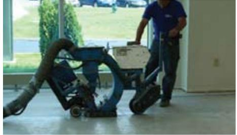
Figure 6.4 – High pressure water wash (water-blasting) will remove the required amount of contaminated concrete. Photo courtesy of Turtleskin, Inc. (protective clothing and gear for use with water blasting) Blastrac® Inc. Shot Blasting Machinery. This method is ideal for preparation of pool tanks, water features and vertical surfaces.
