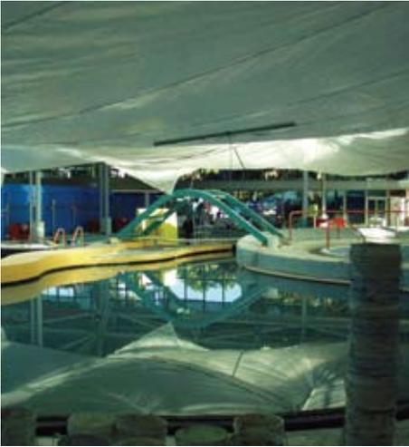
**Case Study 10** – The swimming pool is now in the flood test stage. The waterproofing membrane must be allowed to reach its full cure prior to flood testing. Full cure will vary by manufacturer and product type. The pool is filled at a rate of 1" (25 mm) per hour. Generally the water level will be continually monitored during the length of the flood test (typically 24 - 72 hours) to determine a vessel's 'water-tightness'. The water is then drained at a rate of 1" (25 mm) per hour.
