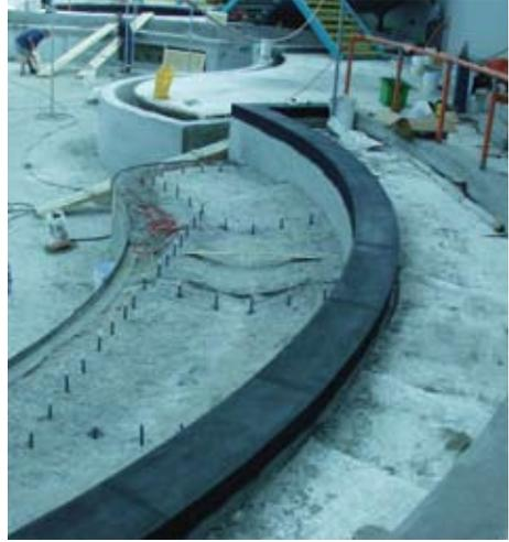
**Case Study 2** – Mechanic is using a wooden template to shape and screed the swale in the water feature tank. Latex fortified portland cement mortars and renders are used for this purpose. Skilled mechanics determine and set finished tile heights, spots, and intersections using lasers, levels and site line builder's transit levels.
