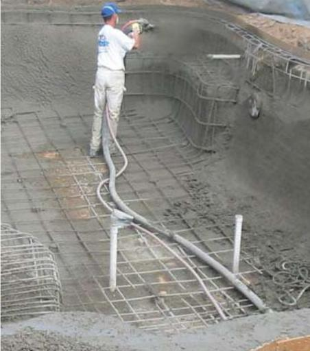
Figure 3.1 – Guniting being sprayed and finished in a residential pool.
