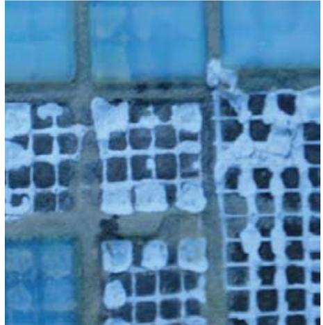
Figure 5.9 – A classic example of an improper adhesive used to mount the mesh for submerged installation. The adhesive has changed color from clear to white and has swelled significantly, forcing delamination.
