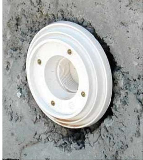
Figure 4.6 – Return port in a concrete shell pool.<sup>7</sup>
