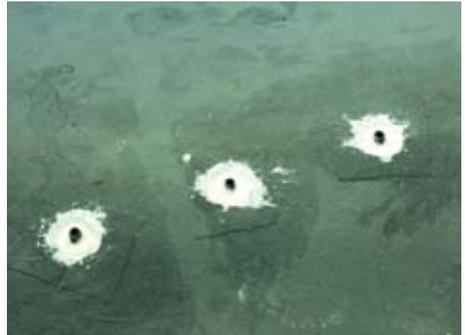
**Case Study 9** – The penetrations are sealed with a suitable flexible sealant. Generally, 100% silicone sealant (e.g. LATICRETE® Latasil™ with LATICRETE 9118 Primer) or urethane sealant with non-solvent based primers can be used. All precautions to create a complete watertight tank must be taken to ensure a successful flood test.
