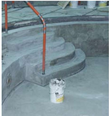
**Case Study 3** – The use of a LATICRETE® liquid latex fortified portland cement based leveling mortar is used to correct any irregularities in the concrete shell. Proper surface preparation will result in an aesthetically pleasing tile or stone finish.
