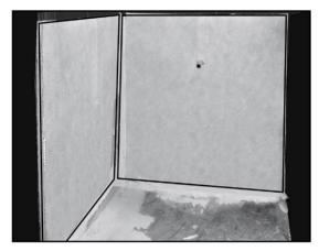
Best practice; sections of HYDRO BAN SHEET MEMBRANE should be butt-jointed and the seam between the HYDRO BAN SHEET MEMBRANE sections should be covered with HYDRO BAN SHEET MEMBRANE Sealing Tape installed with the appropriate thin-set. Make sure that the HYDRO BAN SHEET MEMBRANE Sealing Tape overlaps each HYDRO BAN SHEET MEMBRANE section by a minimum of 2" (5 cm). The floor should be the last section installed.
