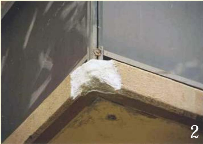
Photo 2: Repair Failure Exhibiting Spalling and Paste Degradation at a Balcony Corner.
