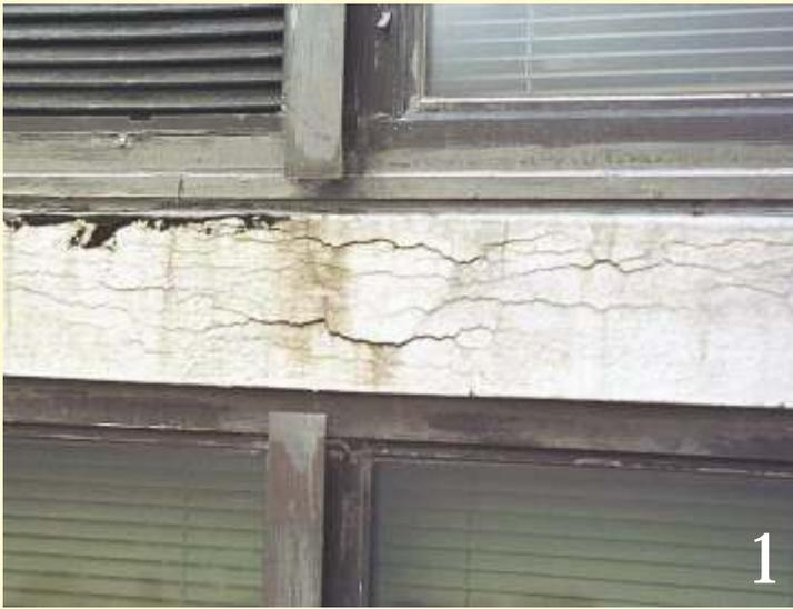
Photo 1: Repair Failure Exhibiting Crack Pattern Indicative of Volumetric Expansion at a Building Slab Edge.
