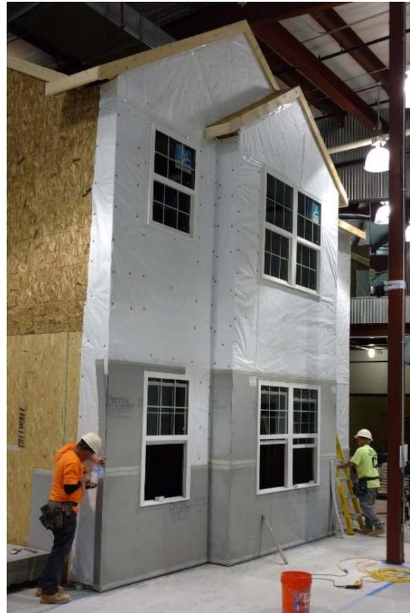
The initial installation was a traditional scratch-and-lath base with Eldorado Stacked Stone veneer, attached with a polymer-modified mortar adhesive. The second installation was National Gypsum’s PermaBase® cement board with Eldorado Stacked Stone veneer attached using LATICRETE® MVIS Veneer Mortar.
