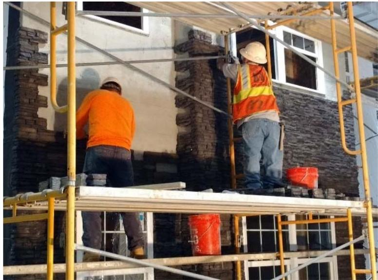
The carpentry crew time savings is related to its members' greater mastery of measuring, cutting, and attaching the cement board (from their experience working with panel products), which suggests that a carpentry crew installing PermaBase® for an adhered veneer base is the most efficient choice.
