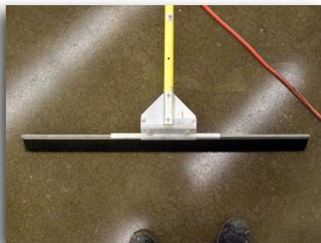
roll (as described above) in the same direction as the broom. Additional ribbons of material should be poured into or added to the existing ribbon of material before it runs dry thus causing the broom to stop. Be certain to always maintain the wet edge. Continue this process across the entire floor.
