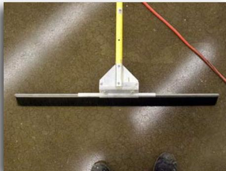
Once the broom is 8-10’ from the starting point begin a perpendicular back roll over that section followed by the finish back roll (as described above) in the same direction as the
