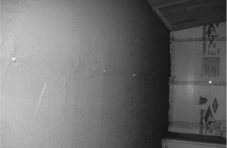
A finished scratch coat wall that is now ready for the float coat.
