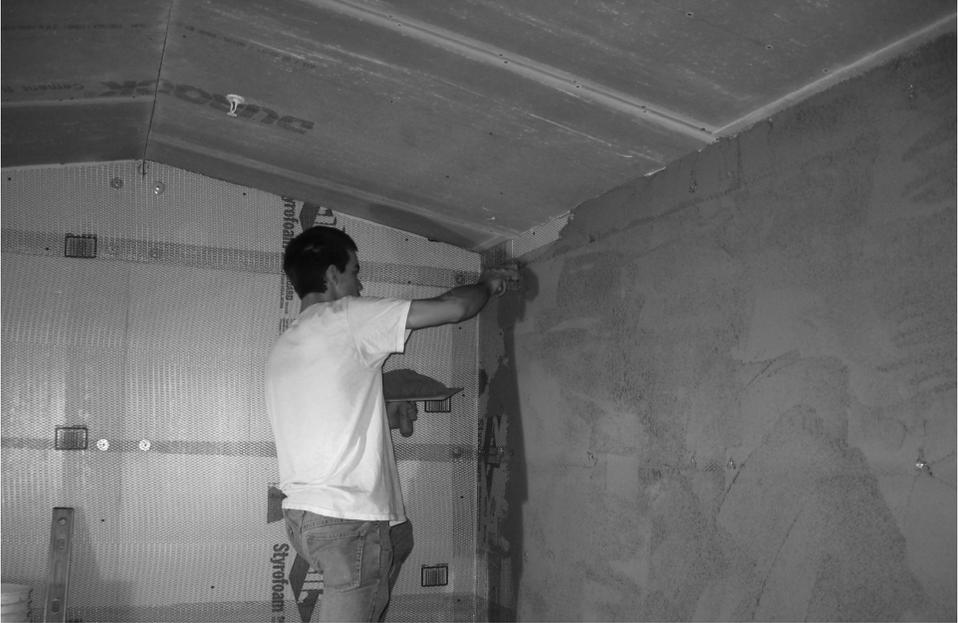
Finishing the application of the 3701 Fortified Mortar Bed scratch coat.
