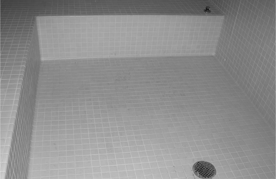
Finished floor installation of tile. Floor and seats are sloped  $\frac{1}{4}$ " per foot (6mm per 300mm) to the drain.
