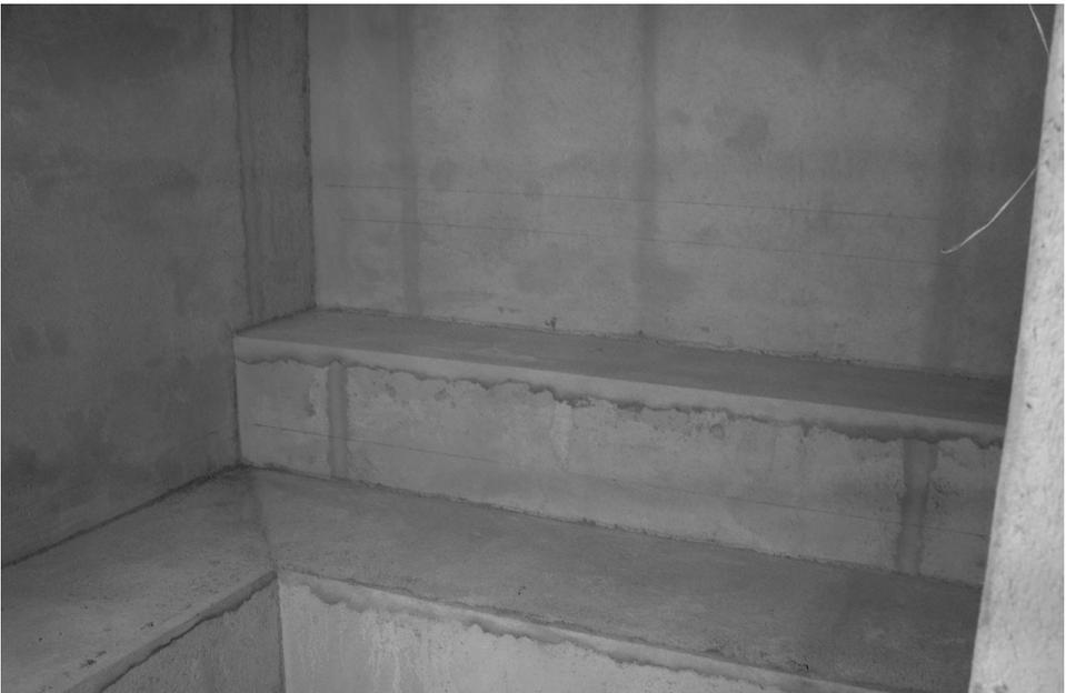
The steam room seats after the installation of the 3701 Fortified Mortar Bed.
