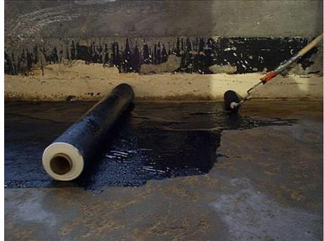
Figure 6.3.6 — 9235 Waterproofing Membrane applied to concrete substrate.
