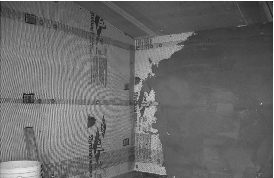
Wall partially finished with scratch coat of 3701 Fortified Mortar Bed.
