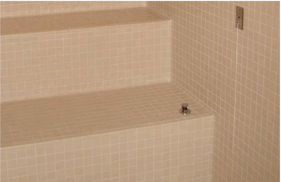
Same view of finished installation after grouting with SPECTRALOCK® PRO Premium Grout and LATASIL™.
