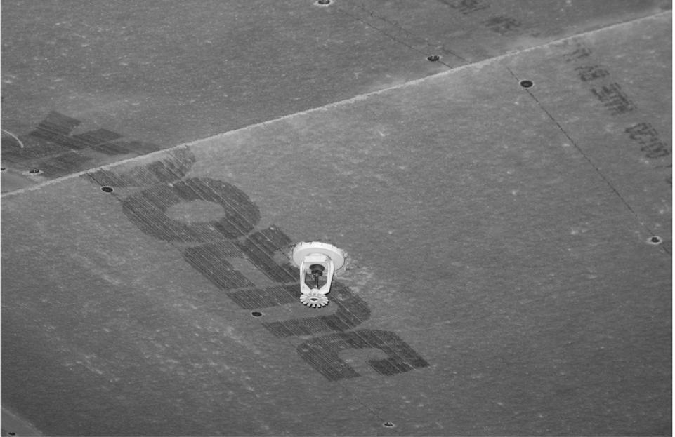
Ceiling (with fire sprinkler head) showing Tile Council of North America (TCNA) recommended pitch of 2" per foot (50mm per 300mm).
