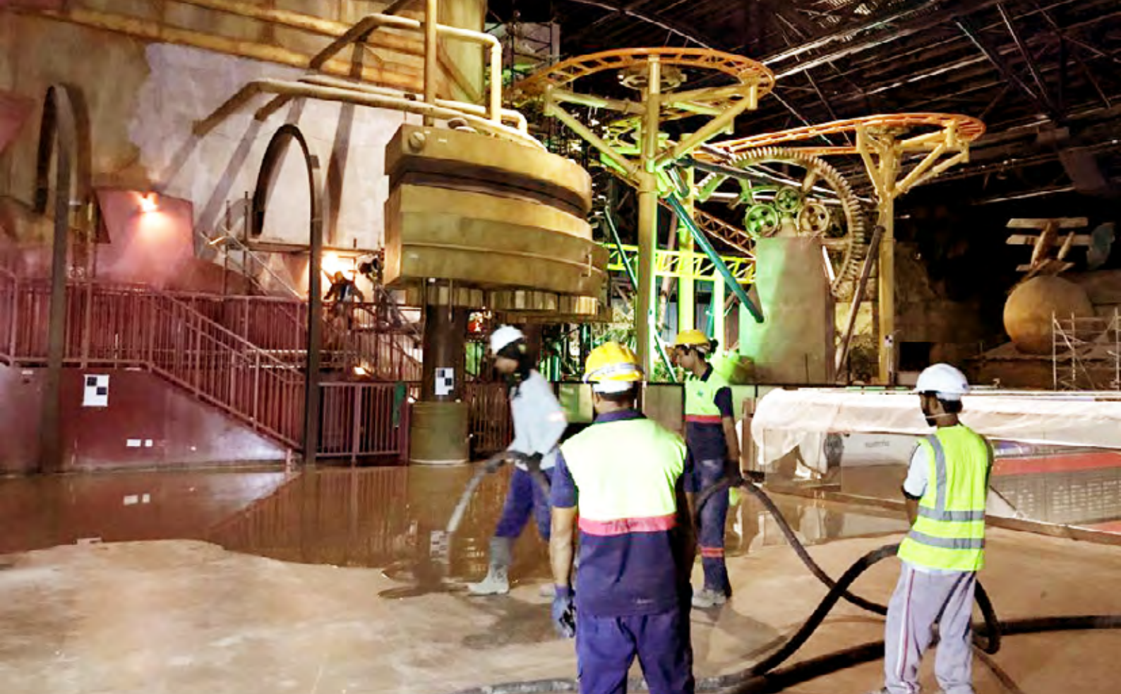
Team LATICRETE pouring self-leveling SUPERCAP SC500 onsite at the Dubai Mall
