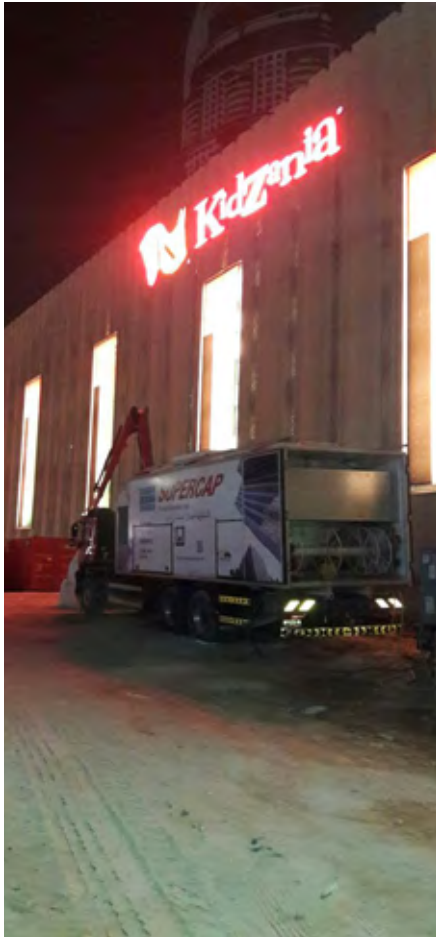
The SUPERCAP Pump Truck onsite at The Dubai Mall
