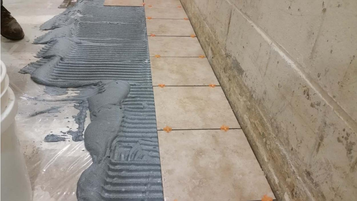
Figure 3 – Mortar and tiles partially installed over concrete slab
