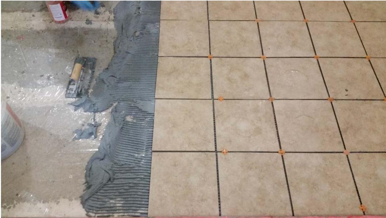
Figure 3 – Mortar and tile partially installed over concrete slab
