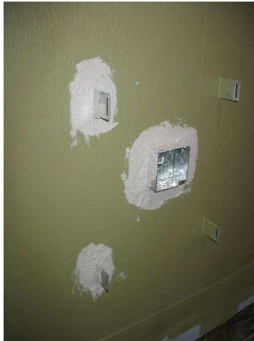
Figure E-10 – Application of LATAPOXY Waterproof Flashing Mortar around Brick Ties and Square Electrical Junction Box / Adjacent Brick Ties Sealed with LATICRETE Air & Water Barrier
