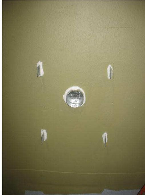
Figure E-11 – Application of MVIS Silicone Sealant around Brick Ties and Hexagonal Electrical Junction Box
