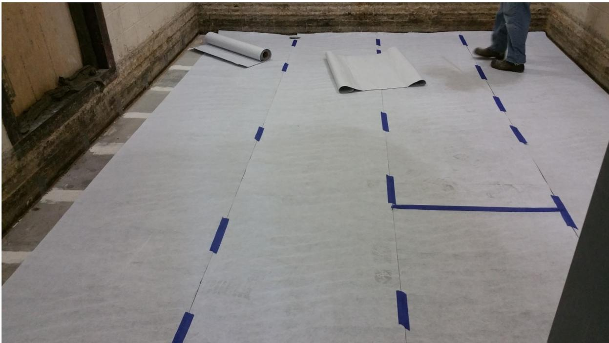
Figure 2 – Fracture Ban™ 90 membrane placed over concrete slabs.
