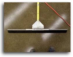
Additional ribbons of material should be poured into or added to the existing ribbon of material before it runs dry thus causing the broom to stop. Be certain to always maintain the wet edge. Continue this process across the entire floor.
