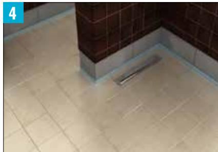
Tiled floors can usually be grouted within 24 hours or the next day. DO NOT switch on the STRATA\_HEAT Wire until the tile adhesive and grout has fully cured. DO NOT use the STRATA\_HEAT Wire to accelerate the drying process of the adhesive.
