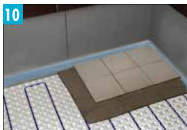
Lay the tiles over the STRATA\_HEAT Mat and Wire. The STRATA\_HEAT Wire, including spliceless connection and termination joint, must be completely encased by the tile adhesive and not exposed. Use PERMACOLOR or SPECTRALOCK grout when grouting
