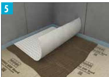
Cut the STRATA\_HEAT Mat to size and press into the adhesive bed using a float or roller, removing any air pockets. Lay additional sheets as above ensuring that the pegs are aligned.
