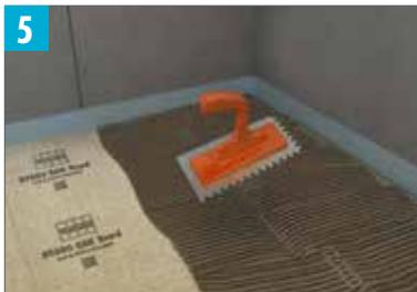
Apply a thin-set layer to the substrate using a  $\frac{1}{4}$ " x  $\frac{1}{4}$ " (6 mm x 6 mm) square notch trowel.
