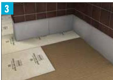
We recommend installing 1/4" (6 mm) HYDRO BAN® Board for optimum performance.
