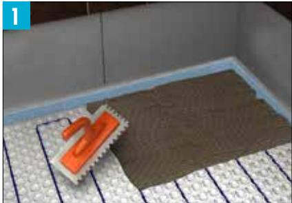
Cover the STRATA\_HEAT™ Mat and Wire with a minimum 1/4" (6 mm) full bed of modified thin-set. Take care not to damage or dislodge the STRATA\_HEAT™ Wire. Do not install tiles smaller than 3 1/2" (89 mm) in length or width.
