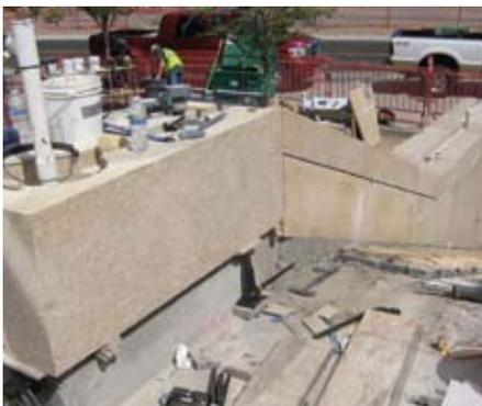
as “very unsettling, but cool,” saw the crane create a problem the stone would later fix itself. At first, the fully-extended crane came up about 6' (1.8 m) short of the distance it needed to make the drop, but in a pleasant turn of events the granite's weight forced the crane to deflect just enough for the stone to be lowered into position.
