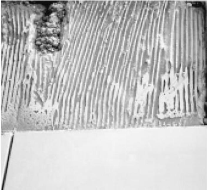
**Picture 1.3 - Insufficient thin set mortar coverage. Removal of a tile reveals many voids that are present in the hardened thin set mortar. Trowel ribbons are inconsistent which will also lead to poor coverage and mortar transfer to the backs of the tiles.**
