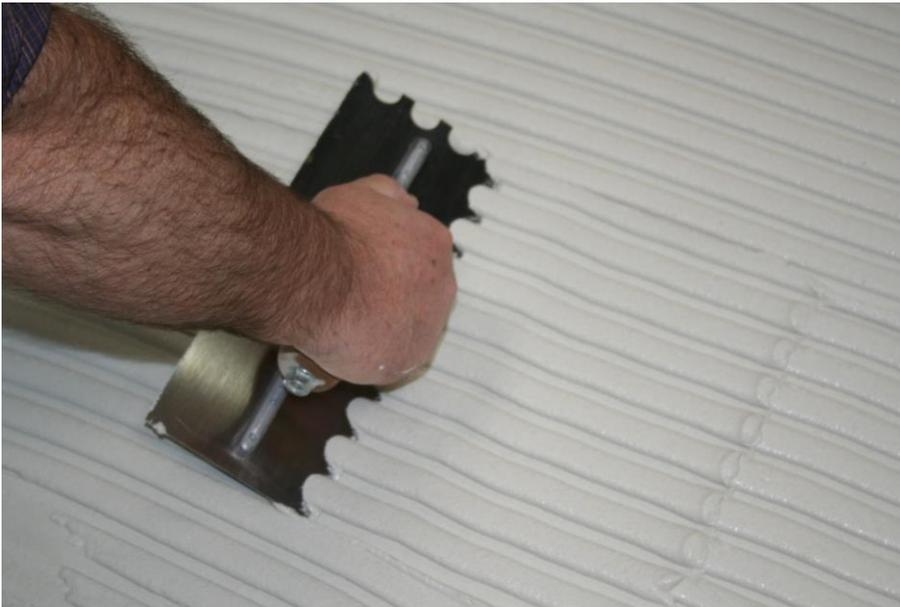
**Picture 1.2 -  $\frac{3}{4}$ " (18mm) loop notch trowel with a medium bed mortar used for large format tiles or stones. Trowel thin set mortar in one direction holding trowel at a 45° angle. Notice the full ribbons of mortar that left behind.**
