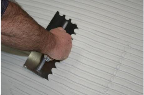
Picture 1.2 - <sup>3</sup>/<sub>4</sub>" (18mm) loop notch trowel with a medium bed mortar used for large format tiles or stones. Trowel thin set mortar in one direction holding trowel at a 45° angle. Notice the full ribbons of mortar that left behind.
