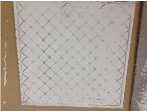
**Figure 1: A properly back buttered large format tile.**
