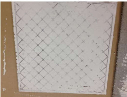
Figure 1: A properly back buttered large format tile.
